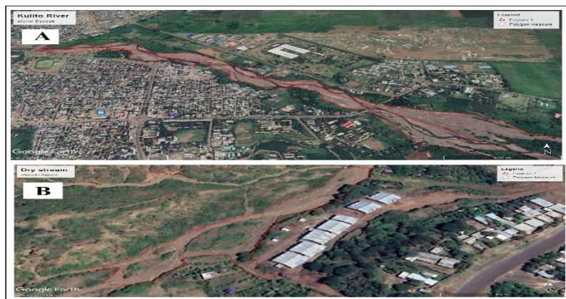
Figure 14 Risk of rapid accumulation of sediments (A) and Risk of Gully erosion and earthflow (B)
