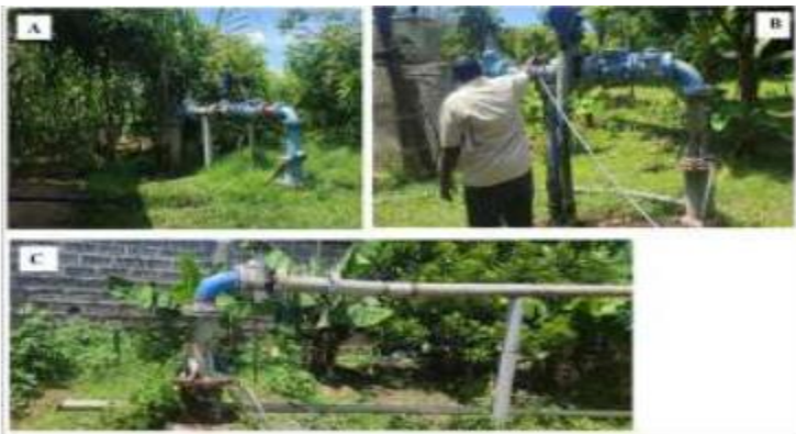
Figure 11 Partial view of sampled boreholes A, Borehole-1 B, Borehole-2 C, Borehole-3
