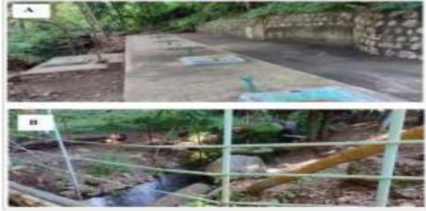
Figure 10 Partial picture of 40 Springs Box (A) and Overflow Springs (B)
